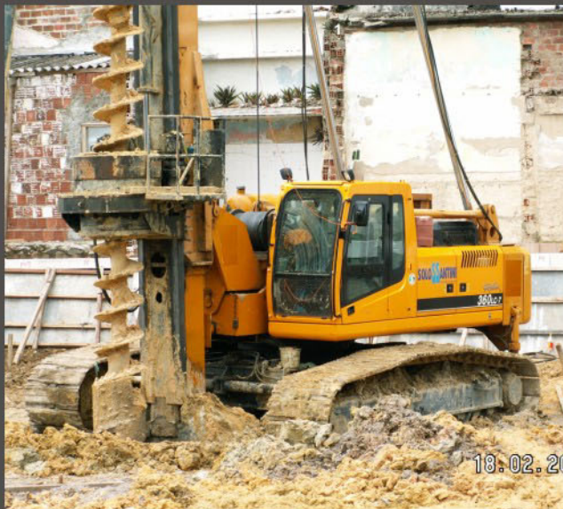
CFA Bottom Drive System
