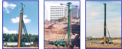
FOUNDATION RIGS AND CRAWLER CRANES
