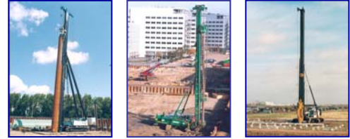
FOUNDATION RIGS AND CRAWLER CRANES
