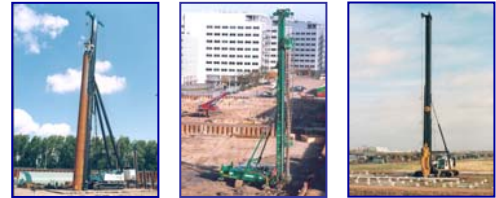
FOUNDATION RIGS AND CRAWLER CRANES
