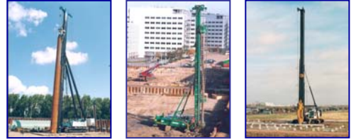
FOUNDATION RIGS AND CRAWLER CRANES
