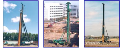
FOUNDATION RIGS AND CRAWLER CRANES
