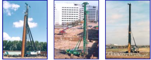
FOUNDATION RIGS AND CRAWLER CRANES
