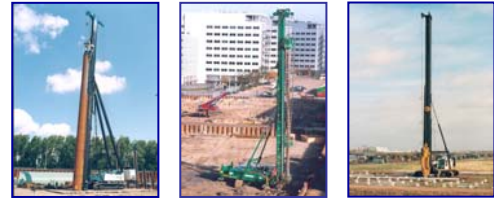
FOUNDATION RIGS AND CRAWLER CRANES
