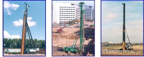
FOUNDATION RIGS AND CRAWLER CRANES
