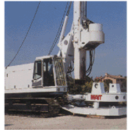
Large bore piles with casing oscillator
