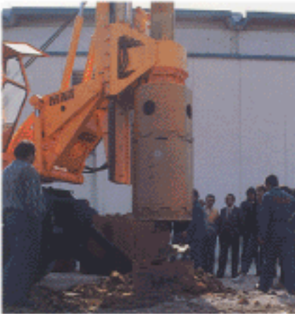
← Drilling with casing tubes
