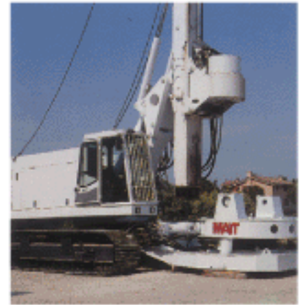
Large bore piles with casing oscillator
