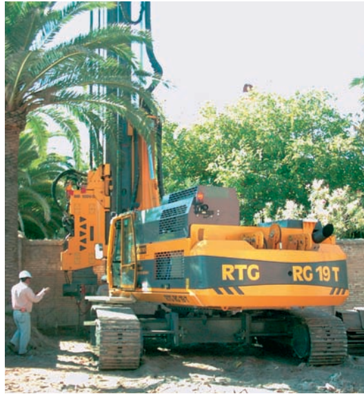
Spundwandeinbau mit Rüttler MR 100V-02 (links oben an RG 19T in Spanien, rechts oben an RG 16T in Dresden) Sheet pile installation with vibrator MR 100V-02 (top left on RG 19T in Spain, top right on RG 16T in Dresden, Germany)
