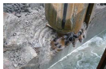
Drilling the existing RC Revetment
