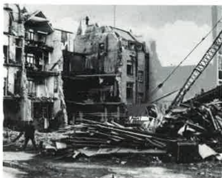
1. Demolition of entire structure.
