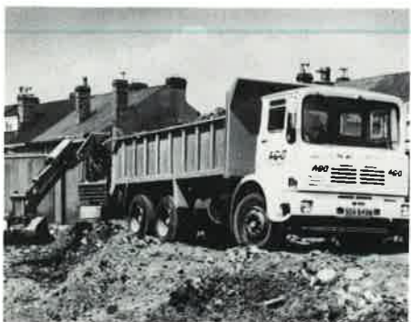
4. Excavation and Site Clearance.
