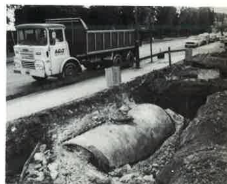
3. Petrol Tank Removal.
