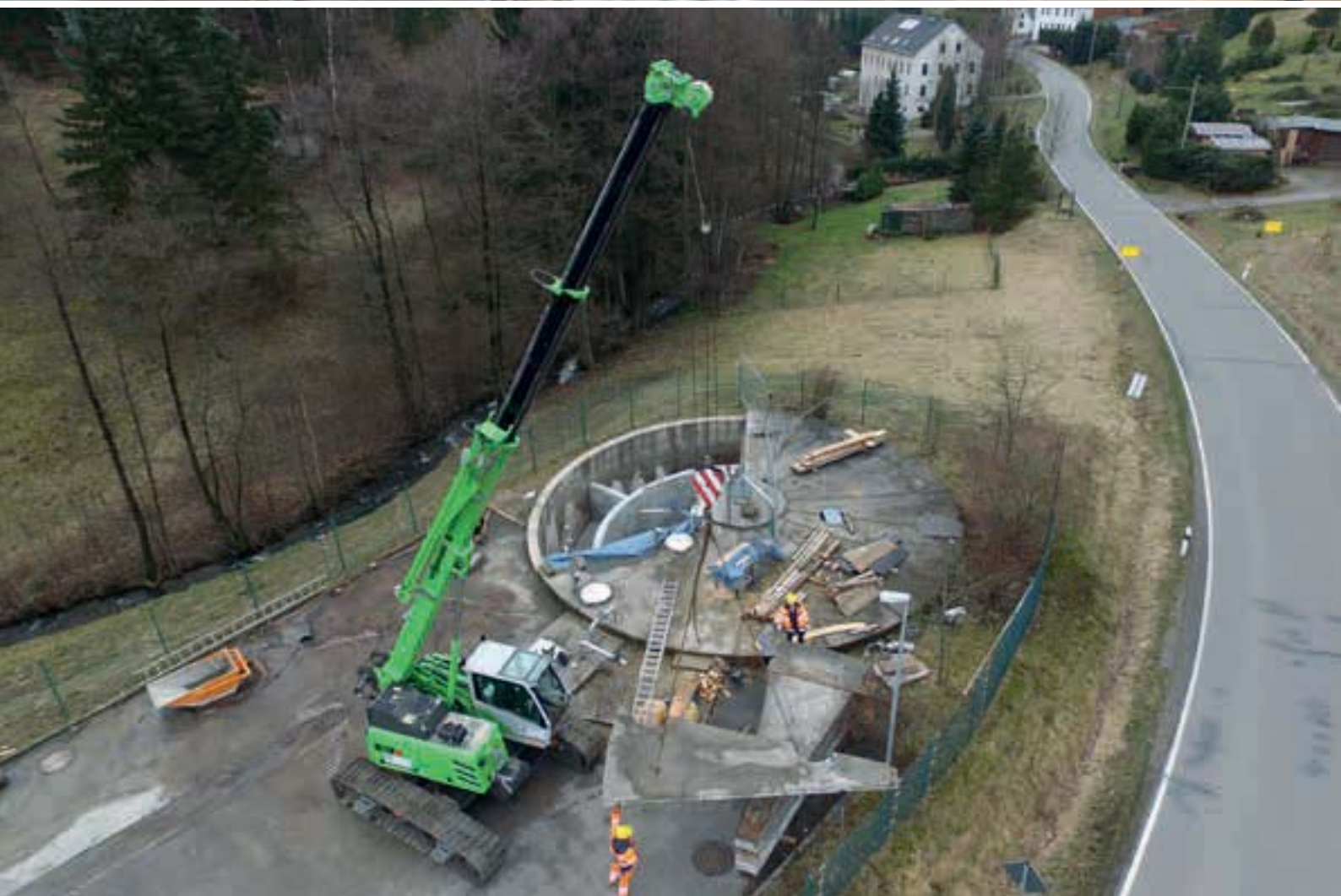
The SENNEBOGEN 613 E crawler crane moves and lifts loads on the construction site of a temporary sewage treatment plant in Germany.
