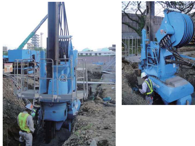
Project : Demolition of Miyagi Prefectural Public Health and Environment Bldg.- Second Phase Location : Sendai City, Miyagi Period : October 2013 ~ November 2013 Silent Piler : F201 Type of Sheet Pile : J Pocket Pile JFESP-4WS, U Sheet Pile SP Ⅱw Pile Length : 4.0 ~ 7.5 m
