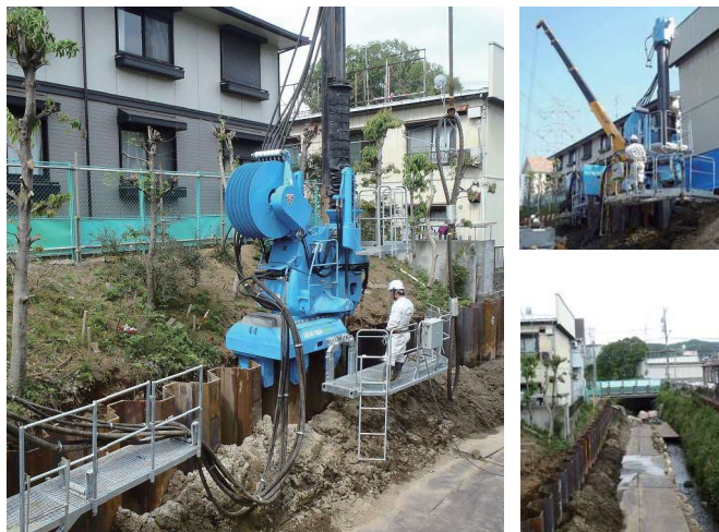
Project : Machida City Public Sewer System, Storm-Water Sewer Construction Works Location : Machida City, Tokyo Period : May 2013 Silent Piler : F201 Type of Sheet Pile : U Sheet Pile SP ⅢL Pile Length : 8.5 m
