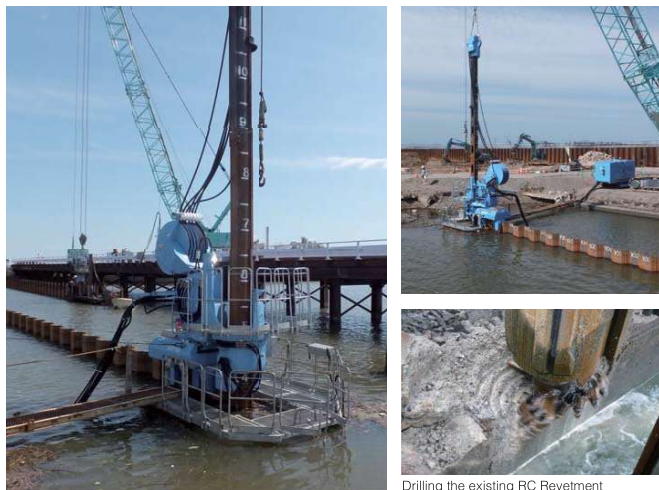
Project : Embankment Restoration Work Section 4, Natori River Location : Natori City, Miyagi Period : September 2013 ~ October 2013 Silent Piler : F201 Type of Sheet Pile : U Sheet Pile SP Ⅲw and SP Ⅳw Pile Length : 7.5 ~ 16.5 m
