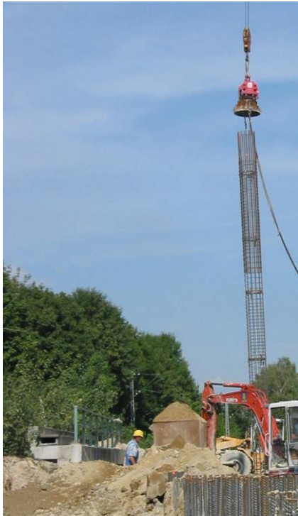
Fig 4: Rebar installation with vibrator
