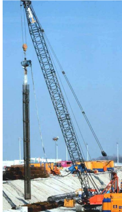
Fig 5: Rebar installation with drawdown beam and vibrator
