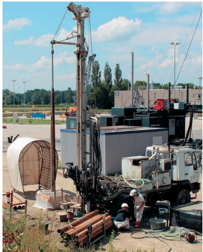
Drilling a vertical core hole with a drilling rig used for exploratory boreholes
