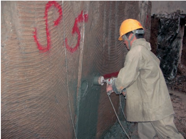
Horizontal core sampling with a hand-held drill
