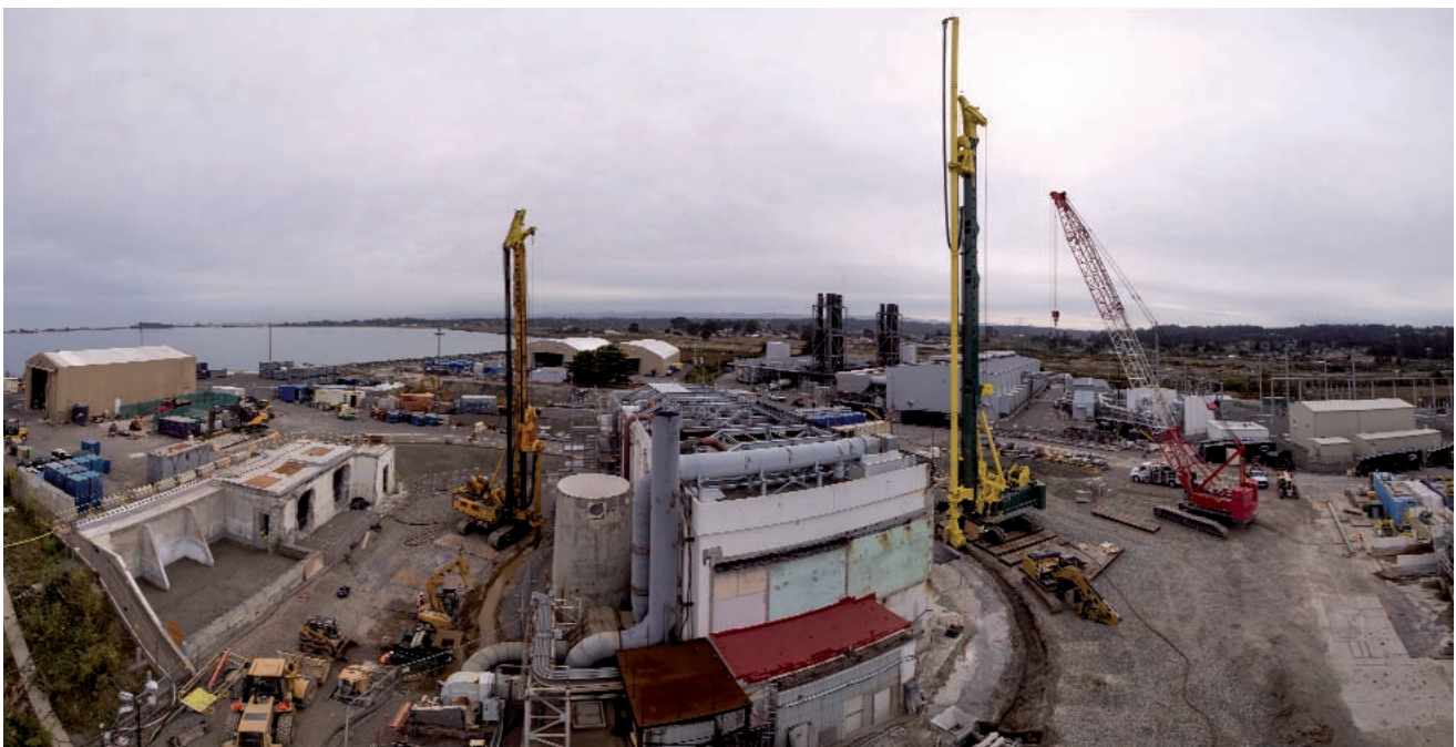
CSM-protection wall around a shut-down nuclear reactor building (USA)
