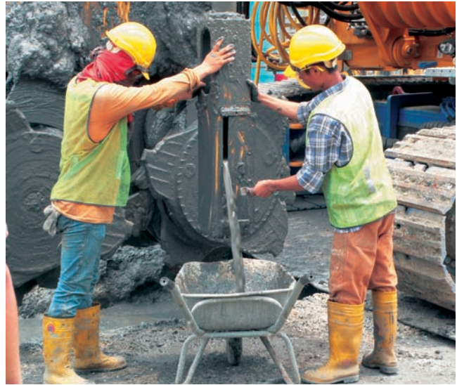
Obtaining fresh samples using a special sampling tool
