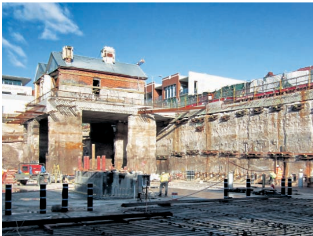
Retaining wall and underpinning for a heritage building with CSM (Australia)
