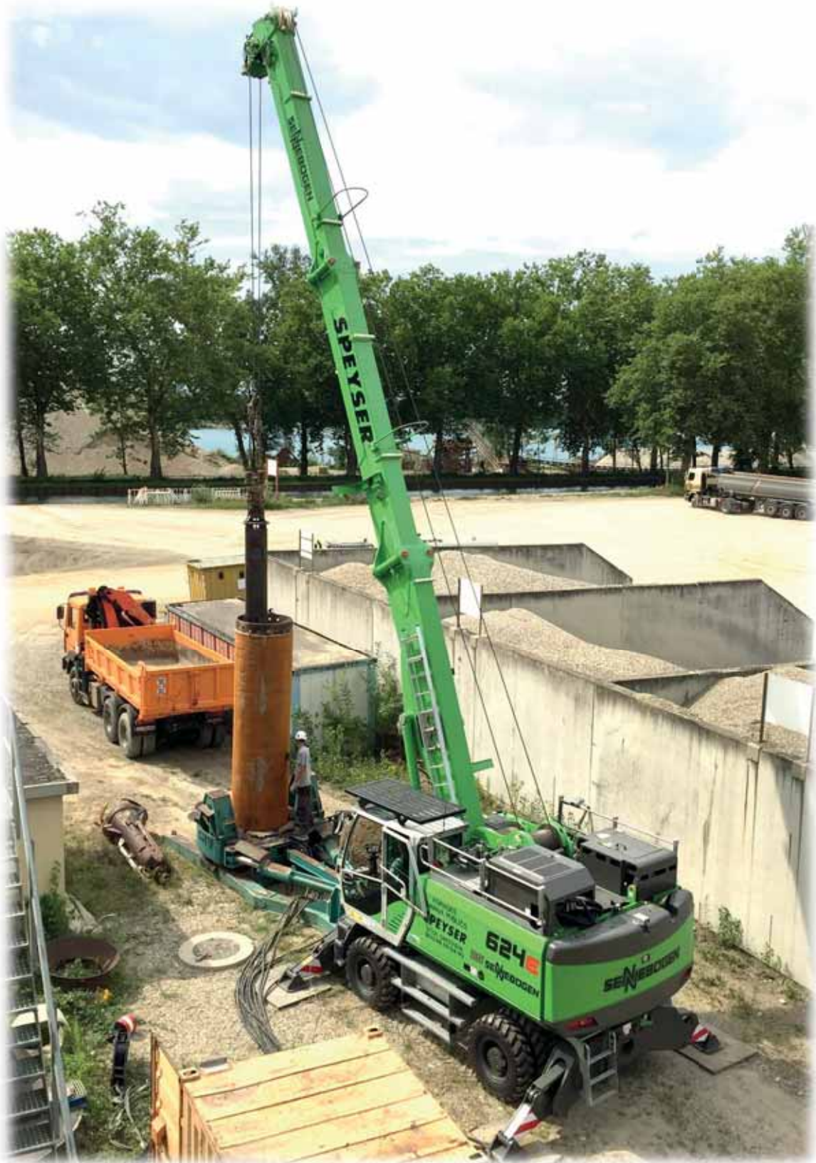
SENNEBOGEN 624HD with casing oscillator – France [source SENNEBOGEN]
