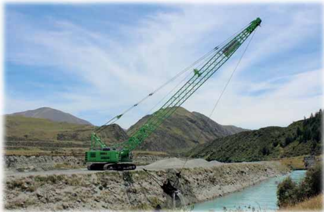
SENNEBOGEN 655HD with dragline bucket – New Zealand [source SENNEBOGEN]
