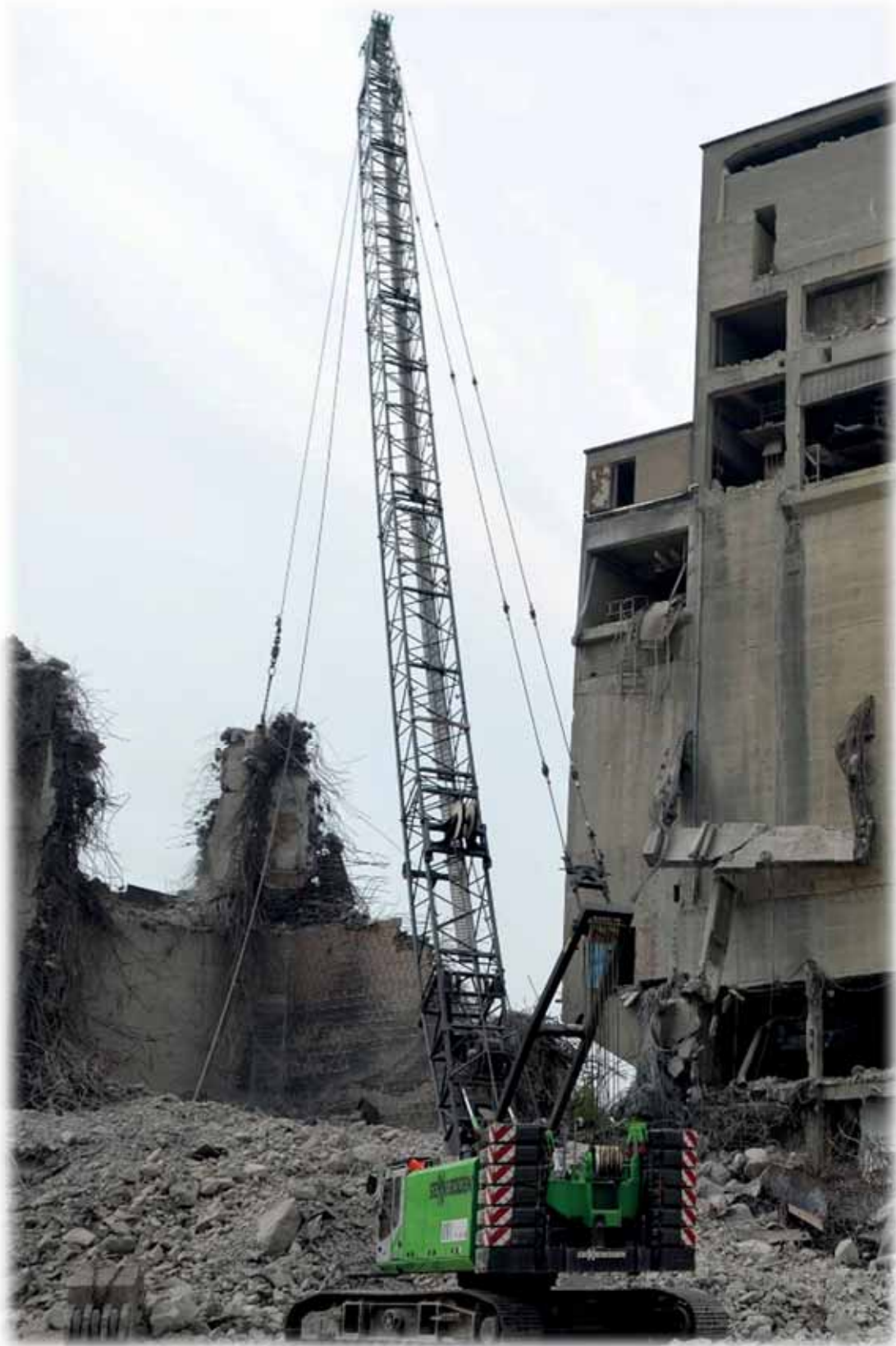
SENNEBOGEN duty cycle crane with wrecking ball in demolition operation
