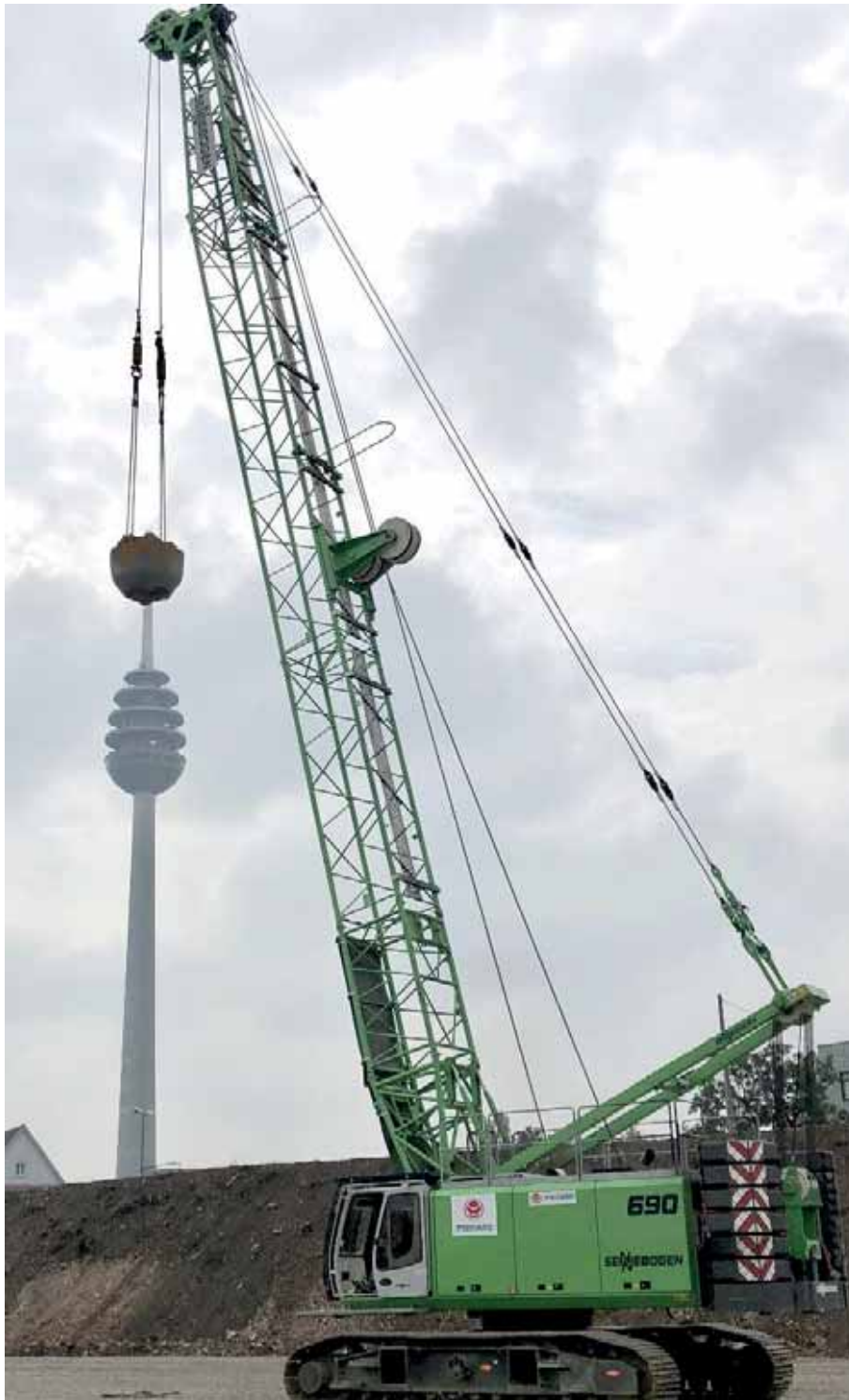
SENNEBOGEN 690HD in dynamic intensive compaction [source: SENNEBOGEN]
