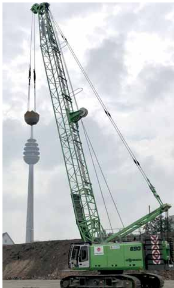
SENNEBOGEN 690HD with drop weight [source SENNEBOGEN]
