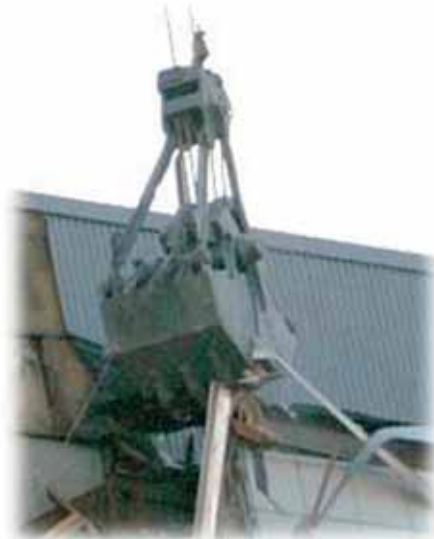
6100HD demolition operation with loading grab [source: SENNEBOGEN]
