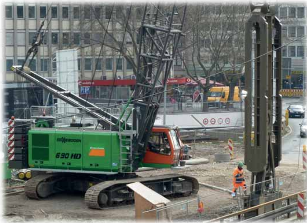
SENNEBOGEN 690HD with mechanical diaphragm wall grab / Germany [source: SENNEBOGEN]
