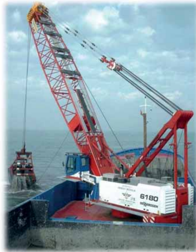
SENNEBOGEN 6180HD stationary on a ship in dredging operation [source: SENNEBOGEN]
