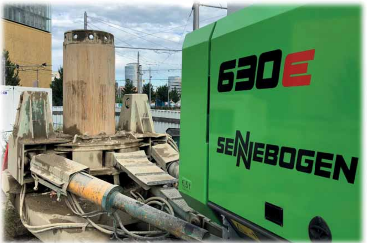
SENNEBOGEN 630HD for grab bores for foundation work [source: SENNEBOGEN]
