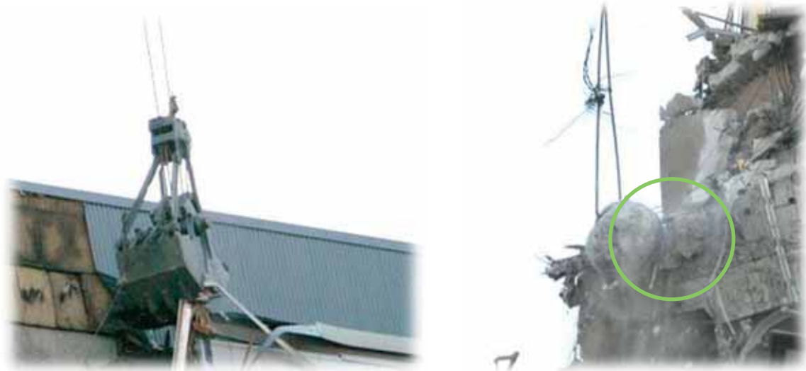
Demolition with rubble grab (left) and wrecking ball (right) [source: SENNEBOGEN]
