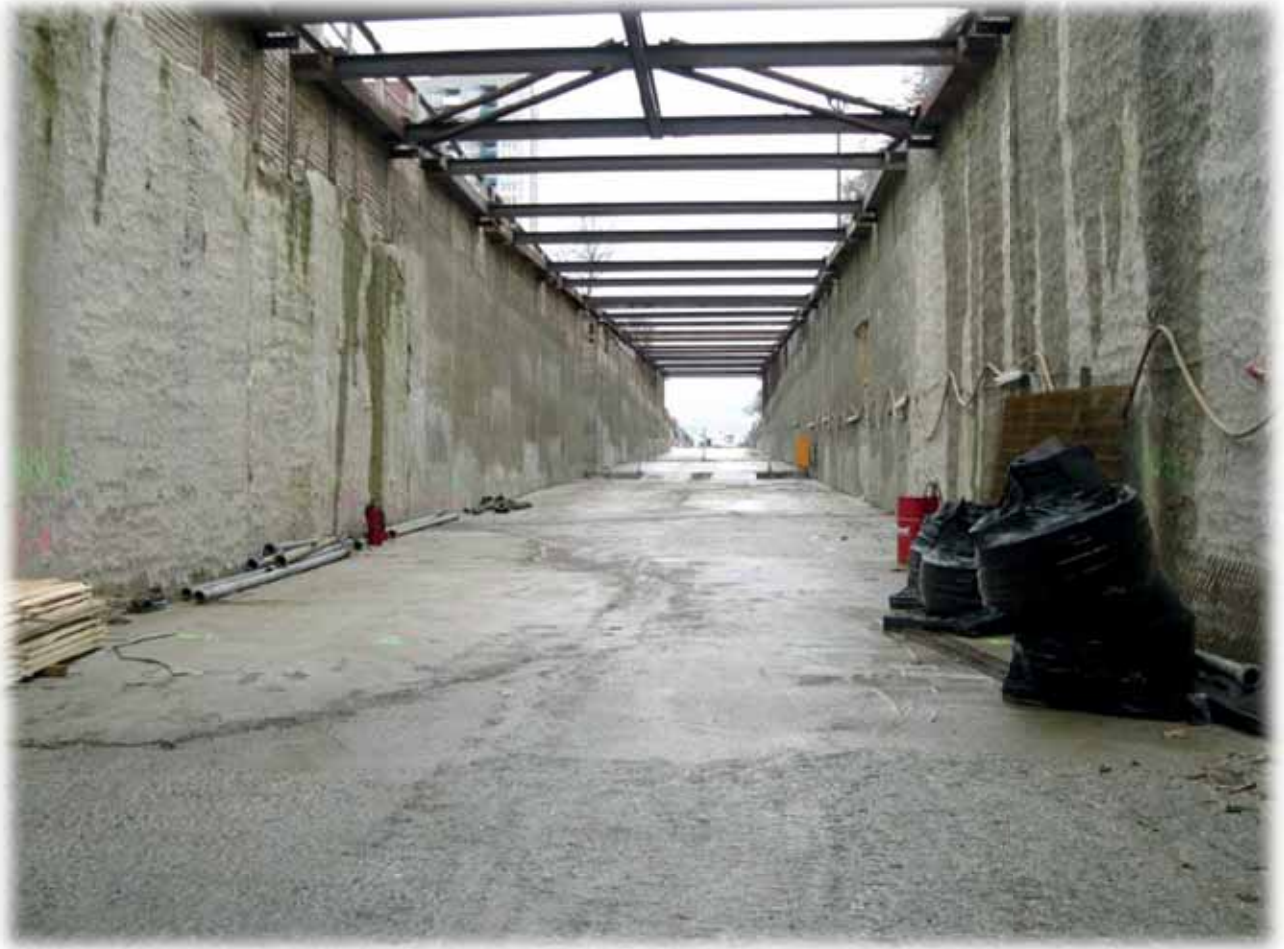
Construction site with diaphragm wall
