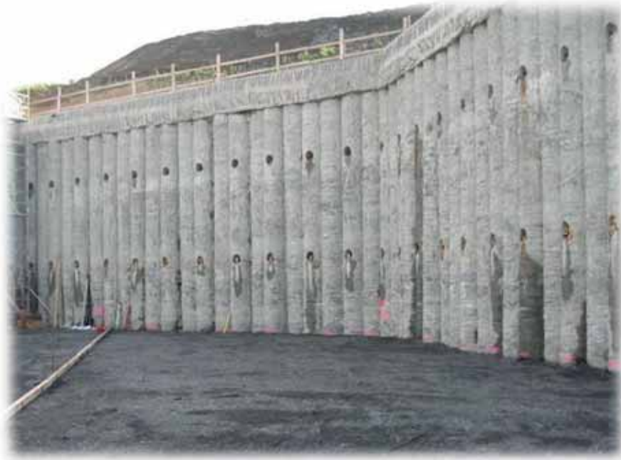
Bored pile wall [source: SENNEBOGEN]
