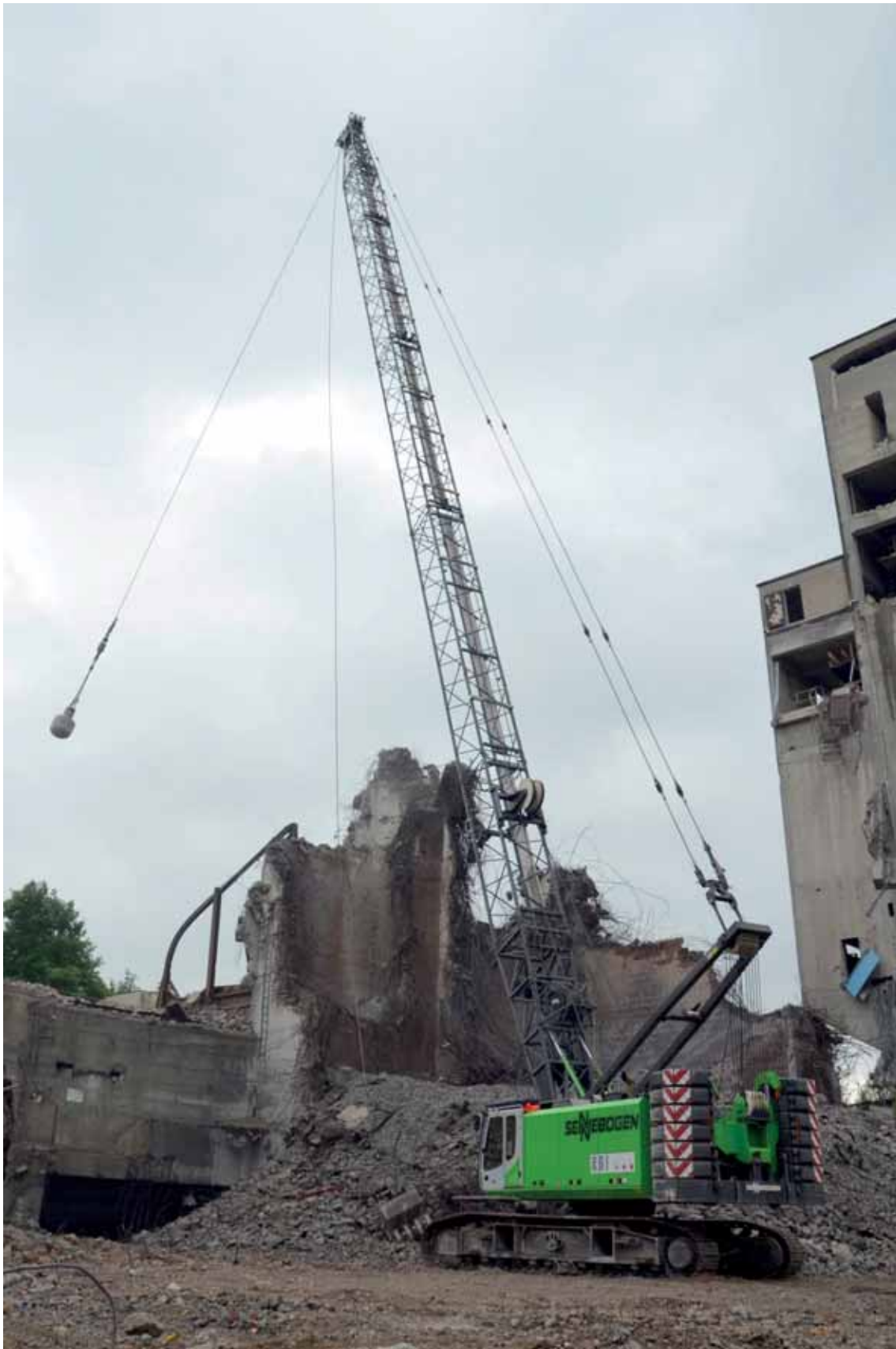
SENNEBOGEN 690HD with wrecking ball / Germany [source SENNEBOGEN]
