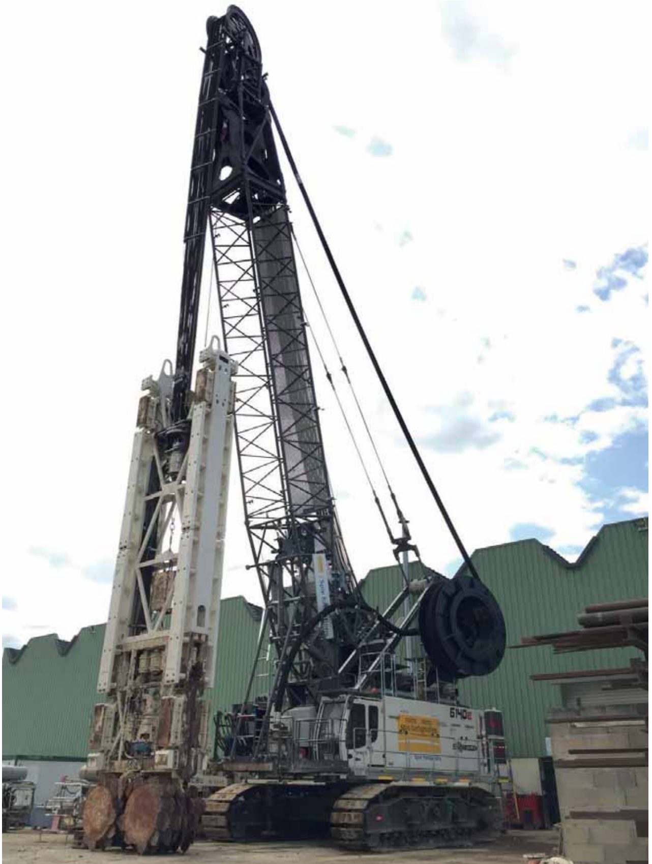
SENNEBOGEN 6140HD (special) with hydromill / France [source SENNEBOGEN]
