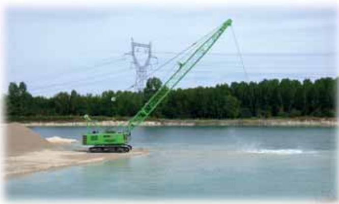
Image 2: Lowering the bucket
