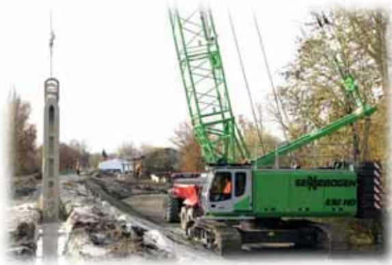
Image 1: Moving grab into the slot
