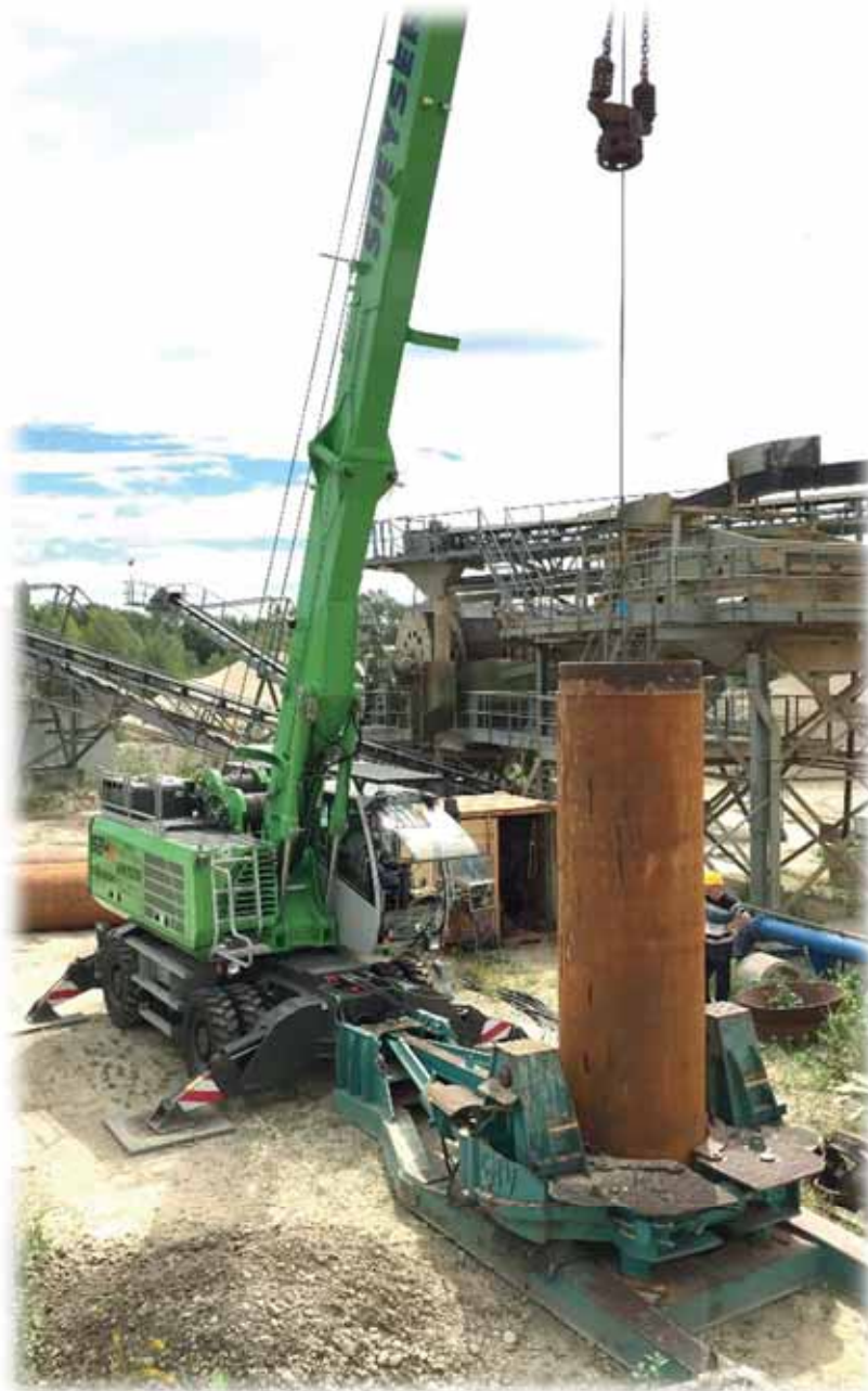
SENNEBOGEN 624HD grab bores in the landfill body [source: SENNEBOGEN]
