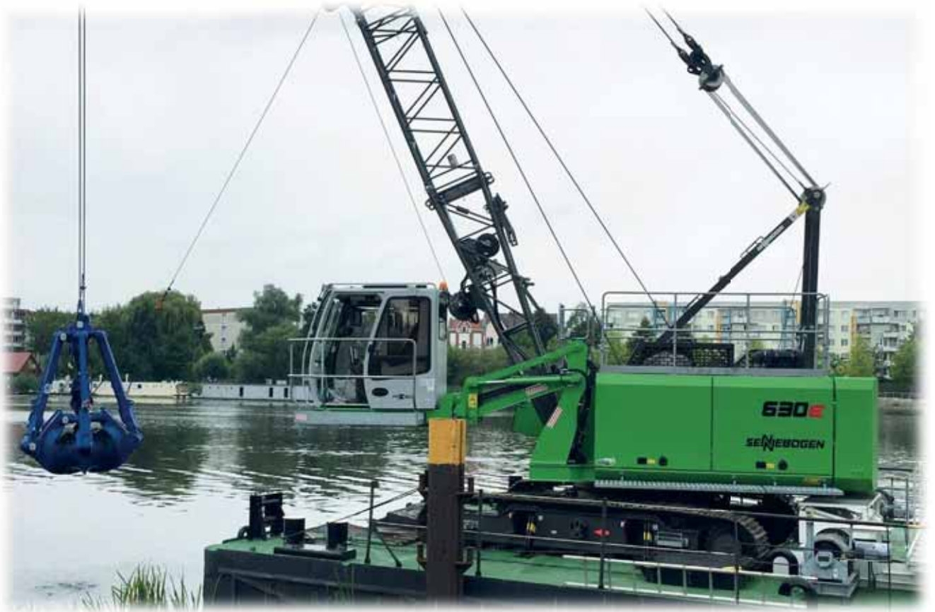
SENNEBOGEN 630HD in grab operation – dredging tasks [source: SENNEBOGEN]
