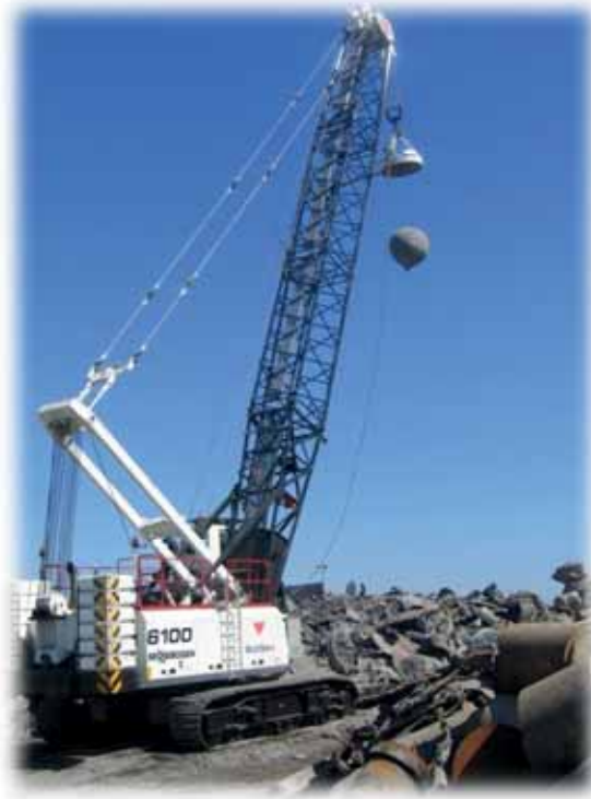
SENNEBOGEN 6100HD diesel engine with double winch, Canada [source MULTISERV Canada]
