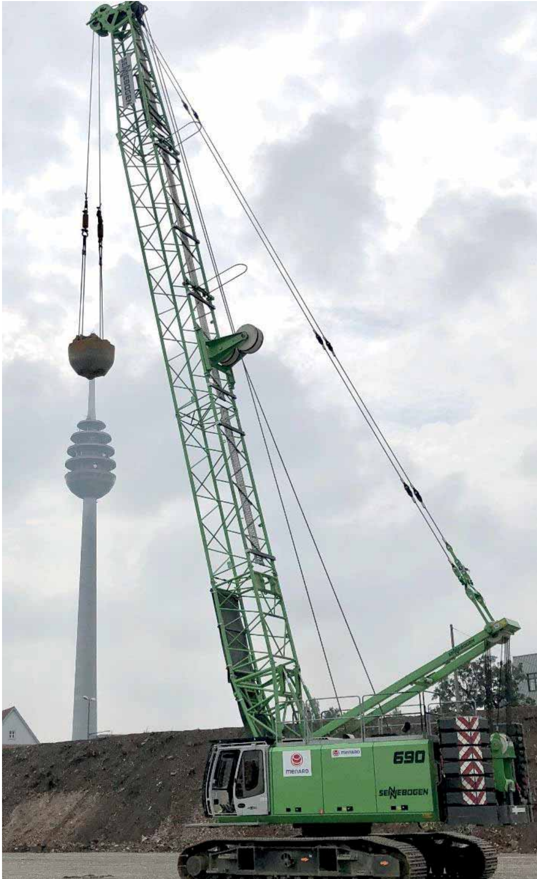
SENNEBOGEN 690 HD deep compaction [source: SENNEBOGEN]
