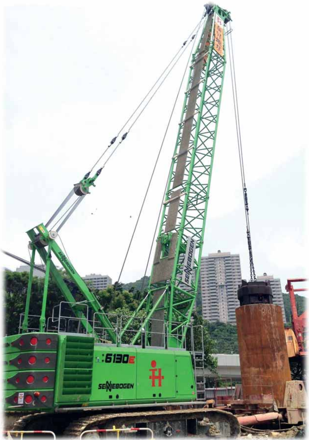
SENNEBOGEN 6130HD with casing oscillator – Hong Kong [source: SENNEBOGEN]
