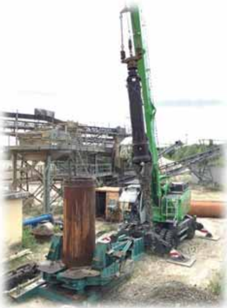
Image 4: Emptying grab and parallel casing installation
