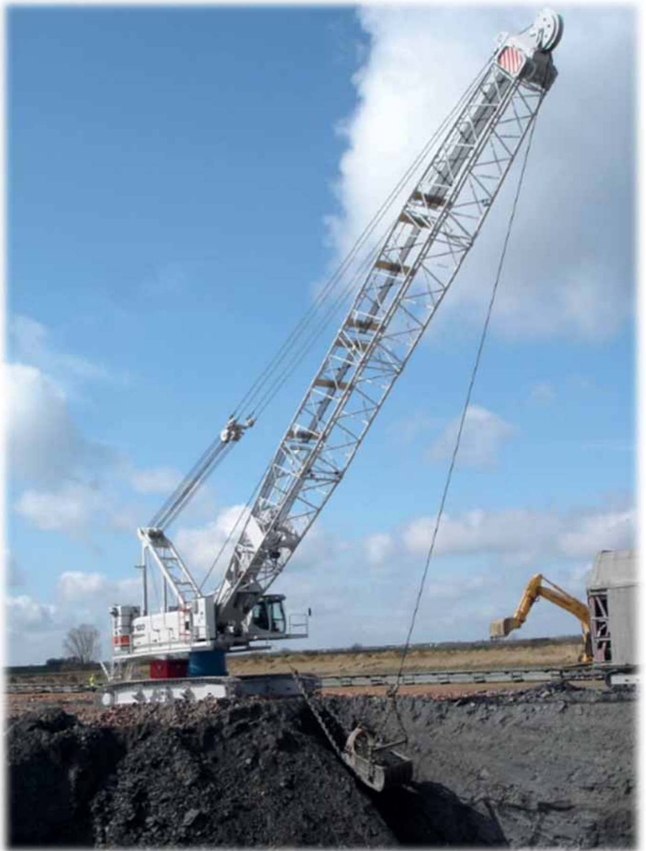
SENNEBOGEN 6180HD in dragline operation [source: SENNEBOGEN]
