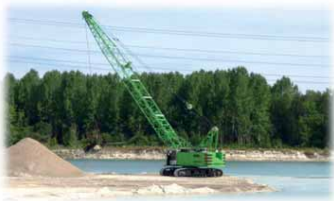
Image 4: Lifting the loaded bucket
