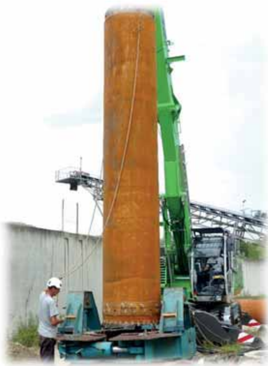
Image 2: Installation of the first pipe section in the casing oscillator
