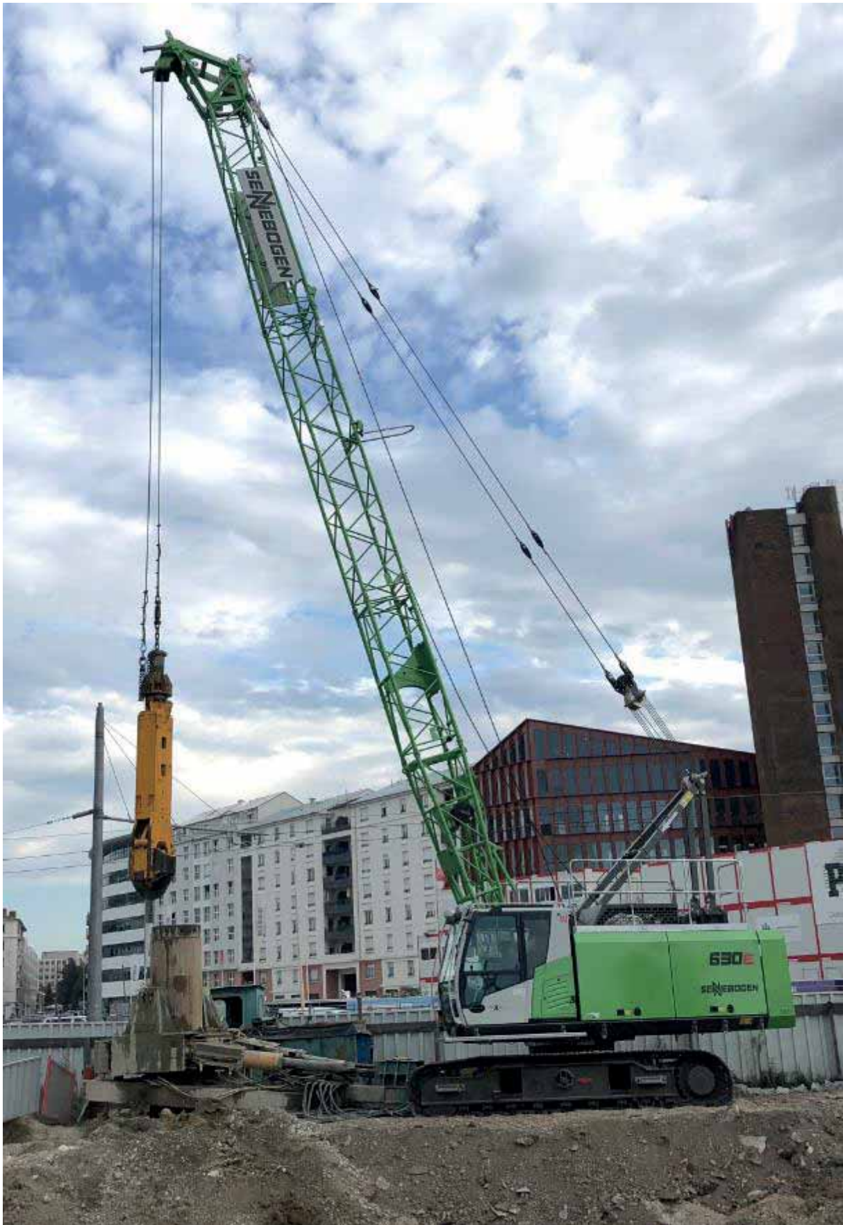
SENNEBOGEN 630HD with casing oscillator – France [source SENNEBOGEN]
