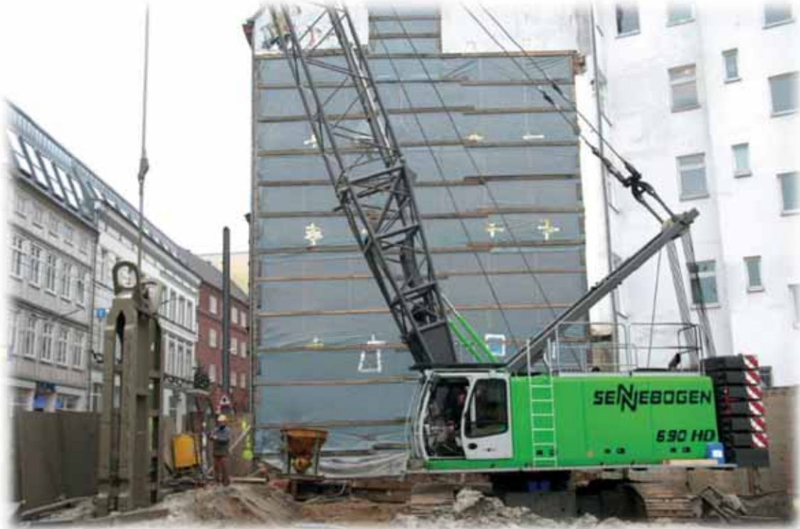
SENNEBOGEN 690HD with mechanical diaphragm wall grab / Germany [source: SENNEBOGEN]
